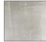
REN-01 Location / North South Walls Product: - Finish: Rendered Colour: Concrete Grey Code: - Note: Render on Concrete fire wall
