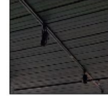
PDC-01 Location / Ceiling Product: Bluescope Steel - Deckform Finish: Powder Coat Colour: Satin Black Code: - Note: Most Likely a Dulux Powdercoat Finish
